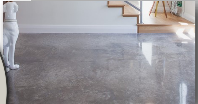
Polished Concrete Flooring Downstairs
